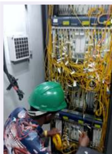
Installation of Optic fibre Distribution Frame (ODF) and Add Drop Multiplexer (ADM) with the configuration and site integration.
