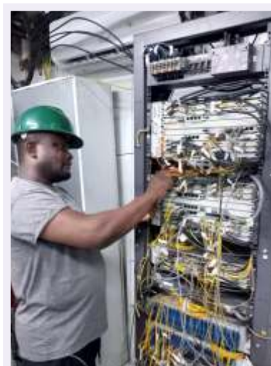
Installation, configuration and commissioning of Mice Wave radios (PDH & SDH)
