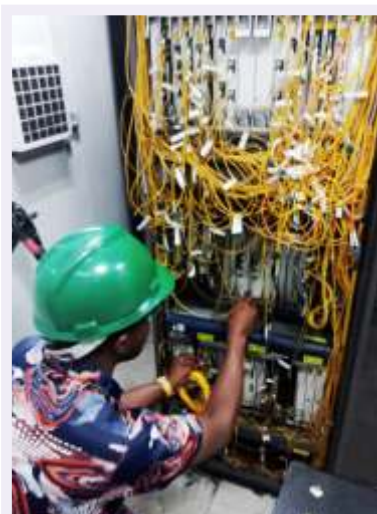
Installation of Optic fibre Distribution Frame (ODF) and Add Drop Multiplexer (ADM) with the configuration and site integration.
